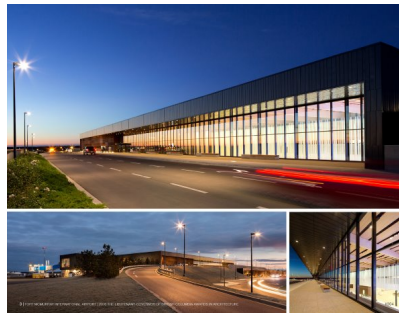
Fort McMurray Airport, International Airport Terminal by mcfarlane biggar architects + designers won in the Lieutenant Governor of British Columbia Awards in Architecture – Merit Level category.
