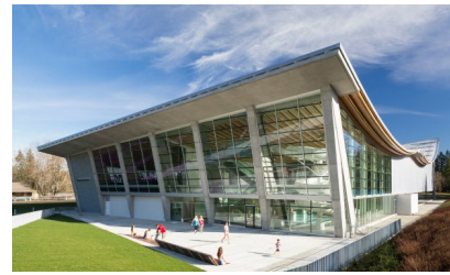
Grandview Heights Aquatic Centre by HCMA Architecture + Design also won in the Lieutenant Governor of British Columbia Awards in Architecture – Merit Level category.
